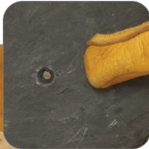
Clean recessed nail holes (as shown)
